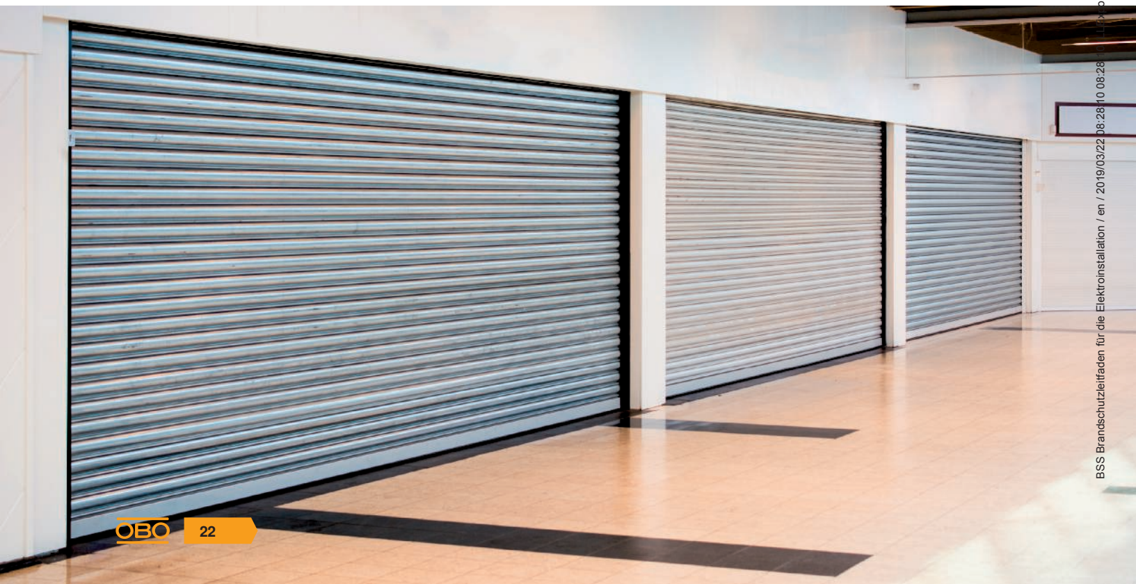
Roller shutters with fire resistance class as fire protection closure
