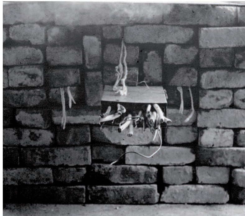
Test structure of the first OBO cable insulation
