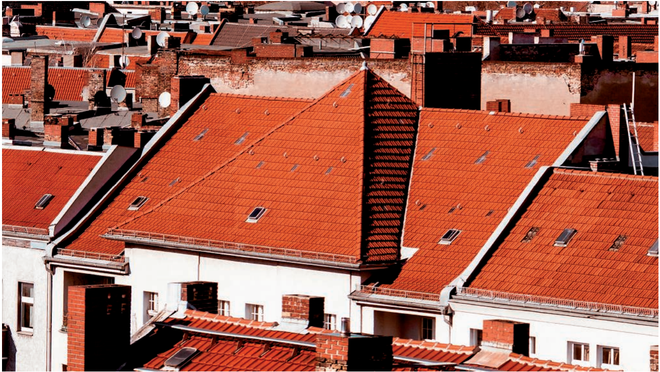
Firewalls prevent the spread of fire
