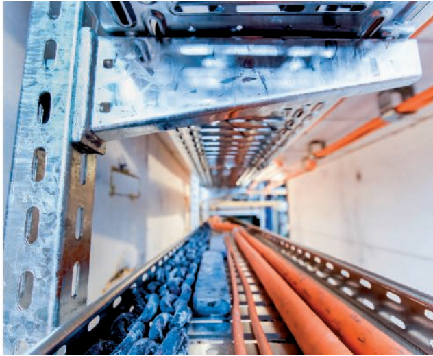
Safety cables before...
