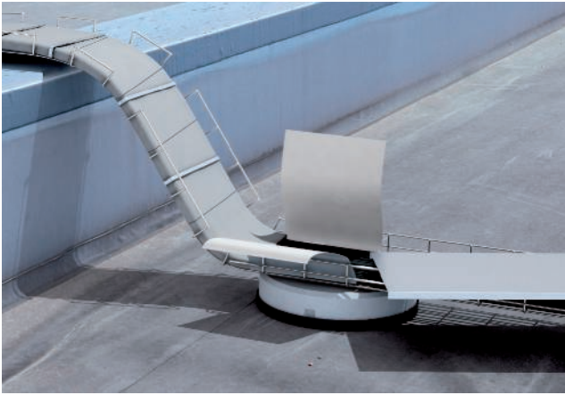
Bandaged cables routed over a firewall
