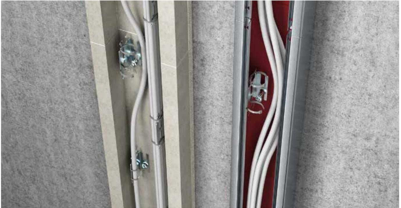
Universal cable bracket for the vertical installation of cables in PYROLINE® Con fire protection ducts made of fibre glass-reinforced, lightweight concrete, as well as PYROLINE® Rapid made of sheet steel with an internal coating.
